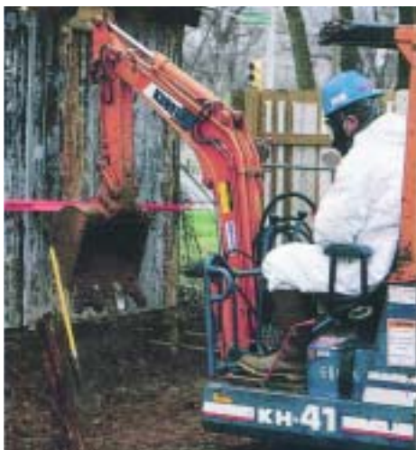
Equipment operators must wear special protective gear when cleaning up contaminated soil.
